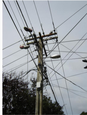
Communication and power lines.
