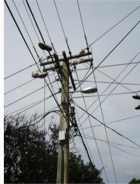
Communication and power lines.
